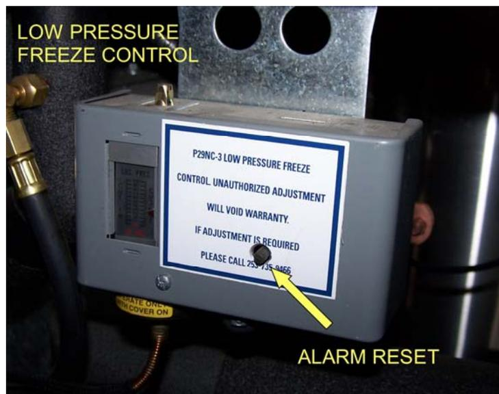
There are many different Freeze or Flow Safety Controls, please refer to the Owner Manual or contact the manufacturer if you are unsure how to reset, or where this control is located.
