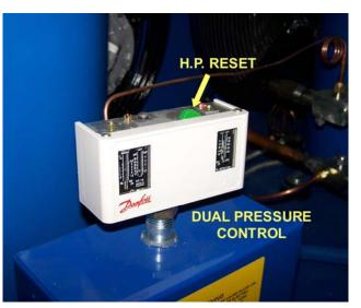
refrigerant pressures have also increased forcing the compressor to operate, momentarily, outside the design envelope. After resetting this control, do not load the system up immediately. It is important that you first drop the glycol temperature in the storage tank to within the design range of the system, before you try to bring your Fermenters back online. When the glycol tank reaches 27 to 35 F, go ahead and start bringing the Fermenters online slowly so as not to overload the system.
