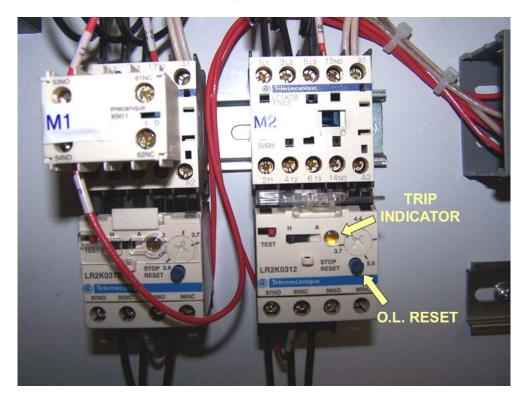
With the control panel open, visually locate the motor starter.
